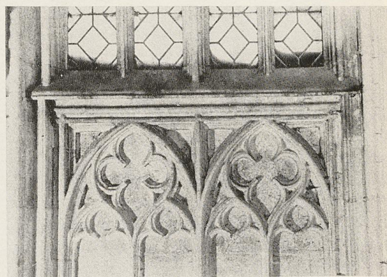
Fig. 3. Bratislava, St. John's Chapel, blind arcade.
