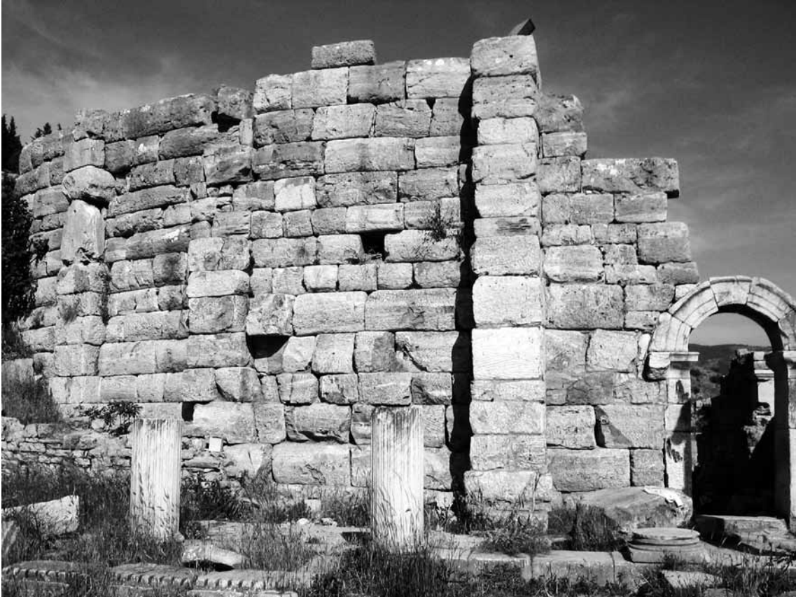
1 Retaining wall of the auditorium , from the west
