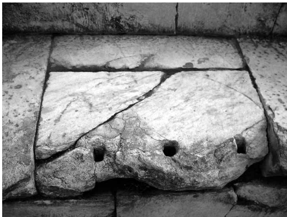
3 Seating slab in row 7, cuneus D, with inscribed circle and dowel holes
