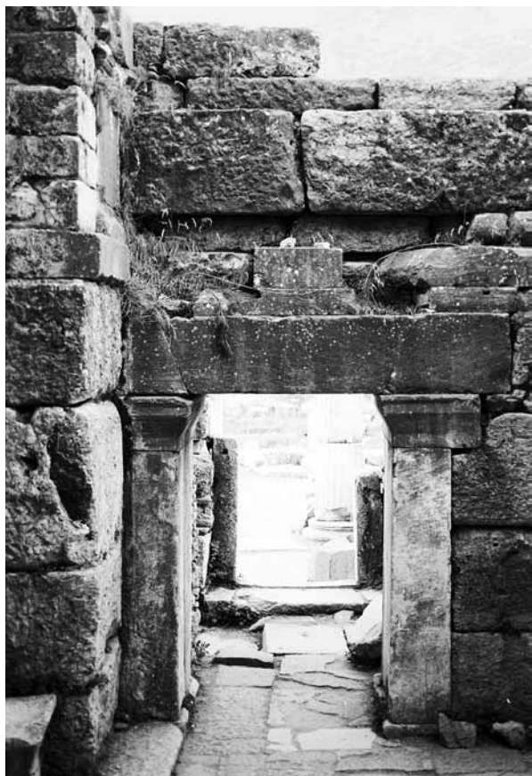
1 Doorway in east parodos from north (SD 7)
