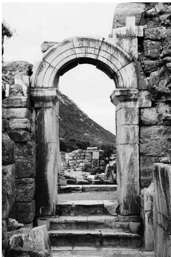
3 Vaulted door in west parodos
