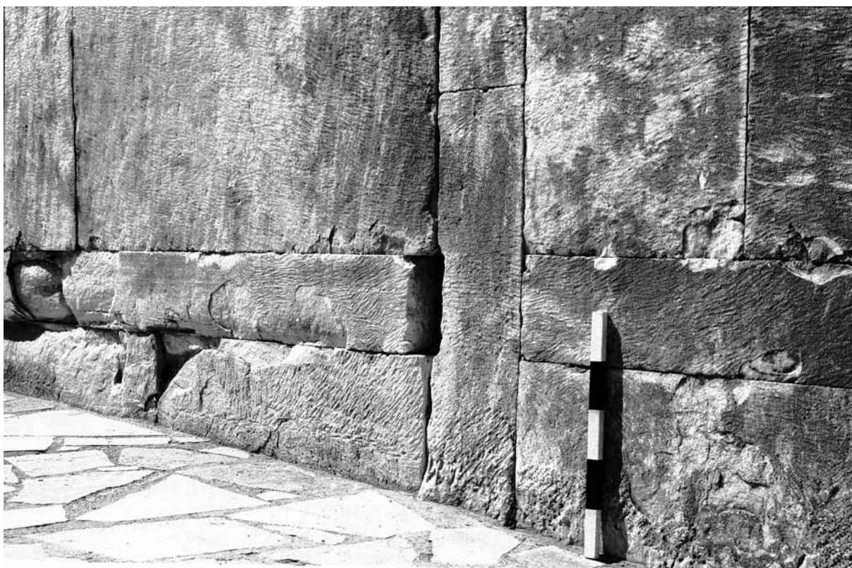
2 Vertical seam in the east analemma wall below the end of the diazoma
