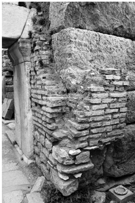
2 Brickwork on the easternmost buttress, next to SD 7
