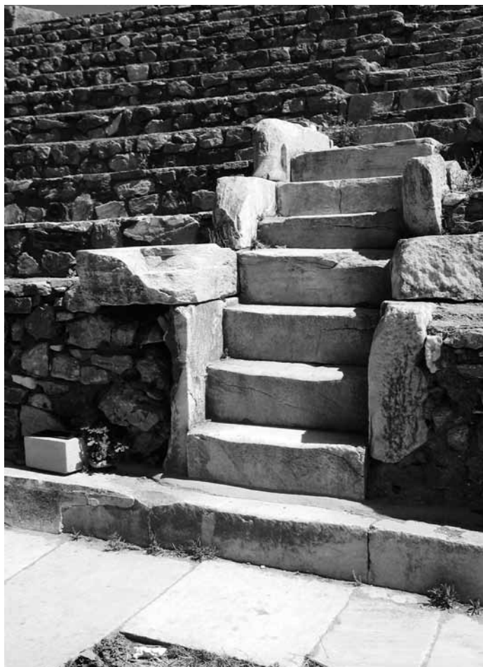
1 Central stairway to the upper diazoma
