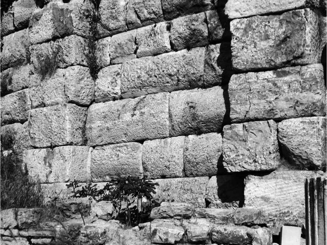
2 Retaining wall, detail between buttress 2 and 3
